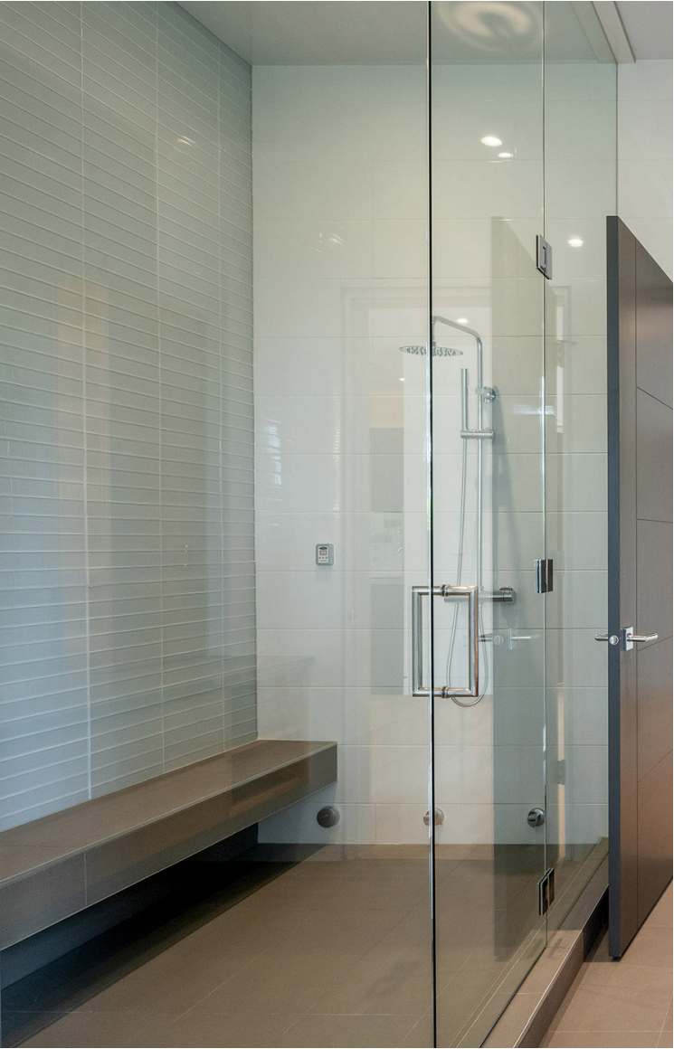
Glass-enclosed steam shower
